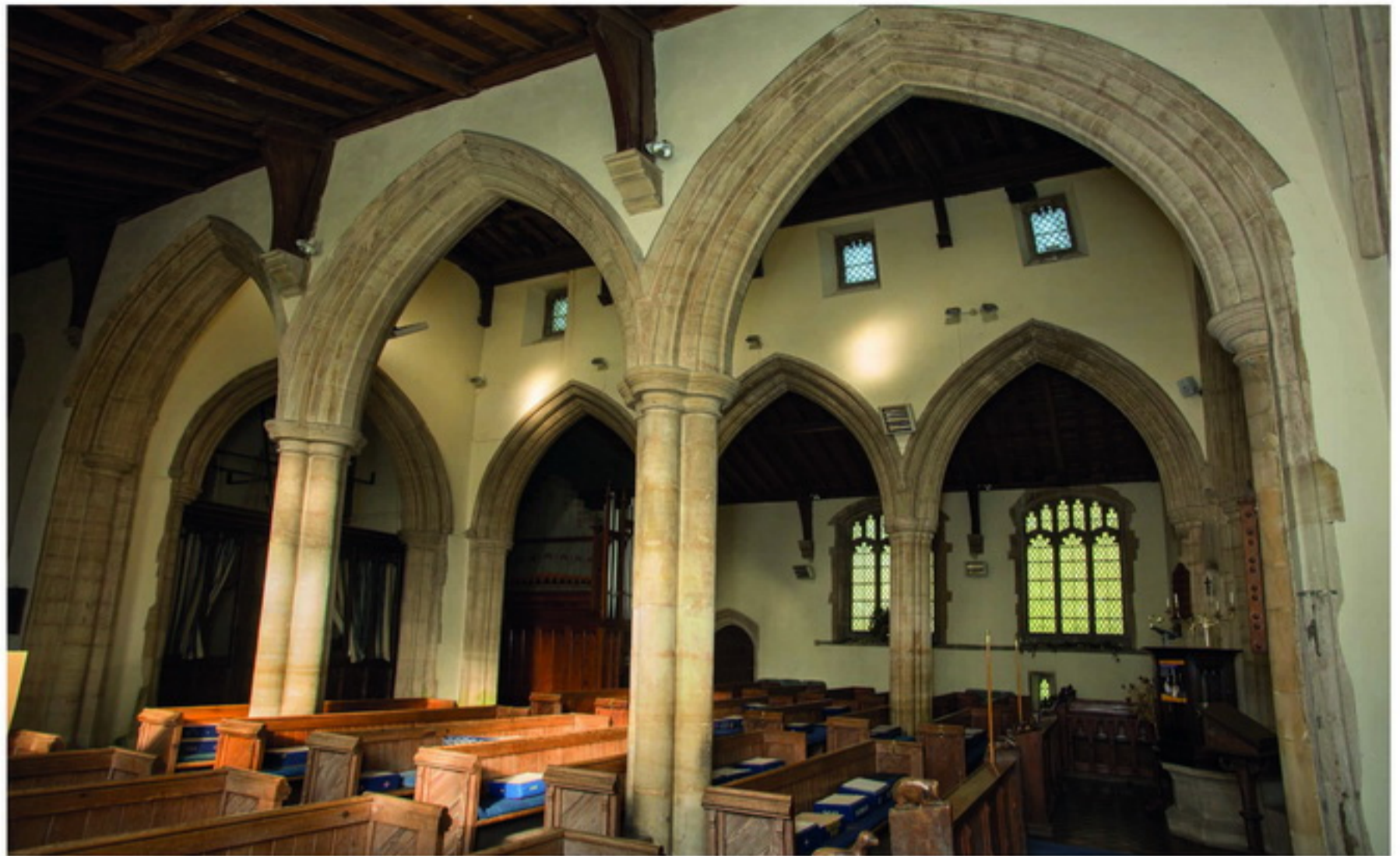
Plate 67 North Aisle viewed through the South Arcade
